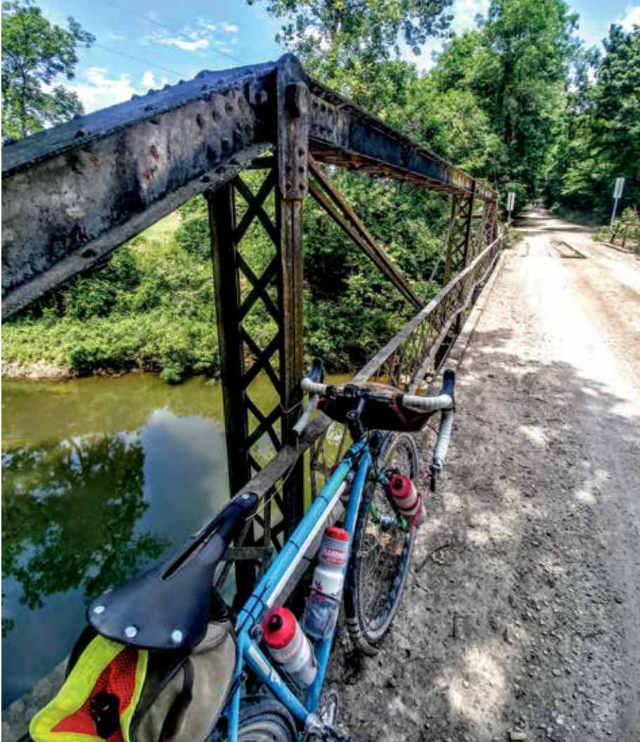
A 110-year-old bridge near Cleveland, MO. —PHOTO KEITH GATES
